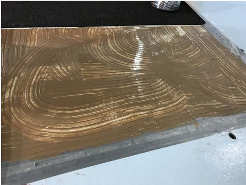
Figure 2.3: adhesive applied to reference floor for underlay
